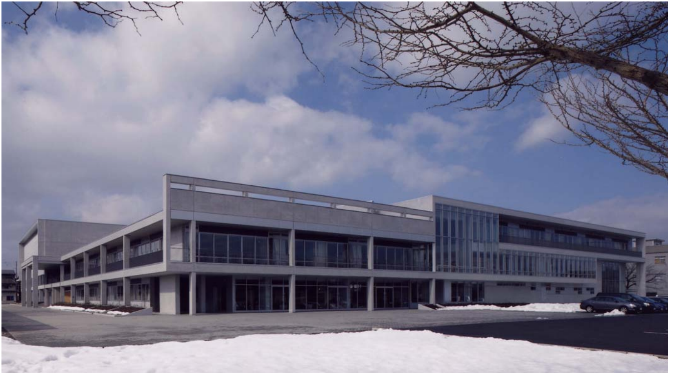
南東側外観 view from southeast
