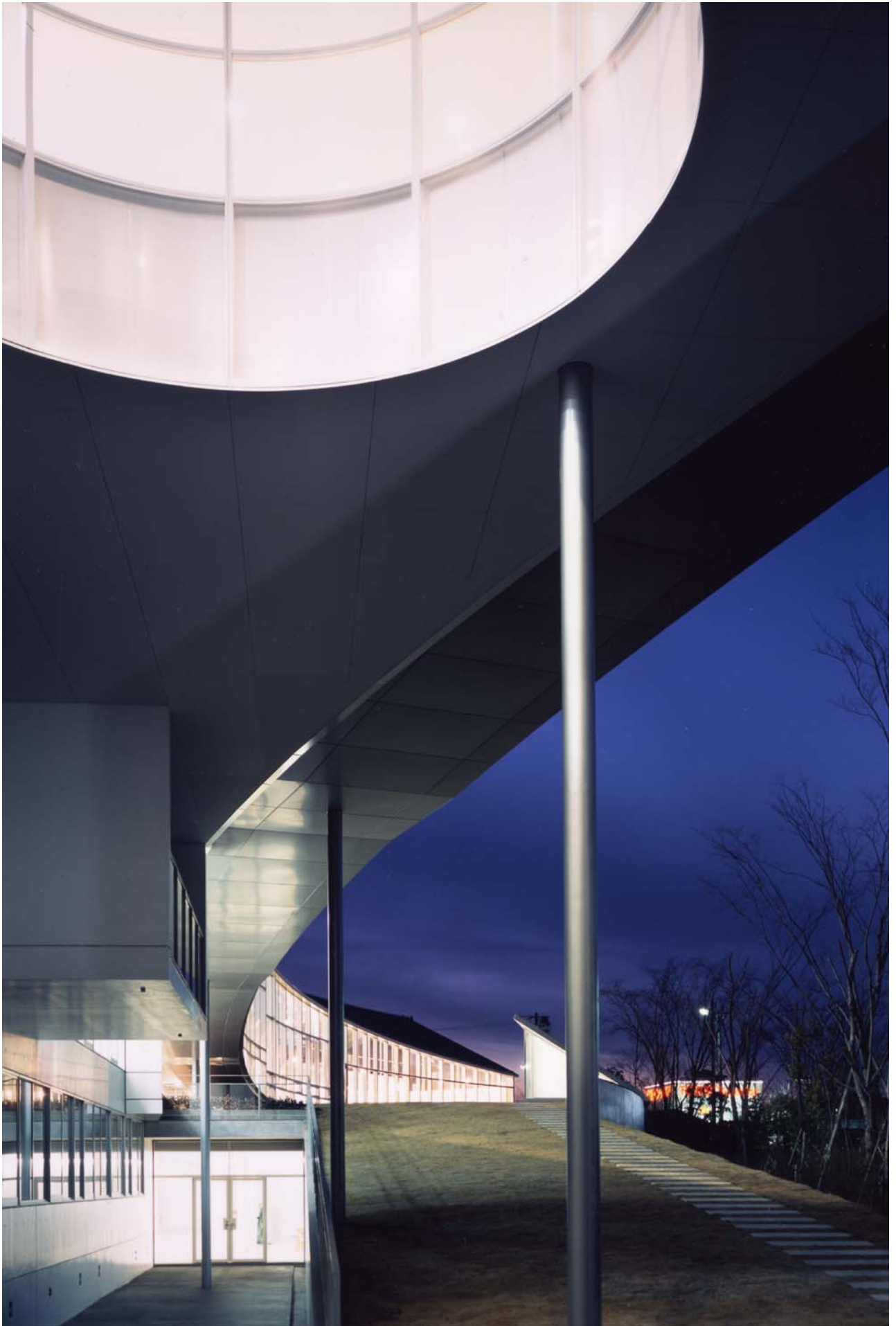
東側外観 view from east
