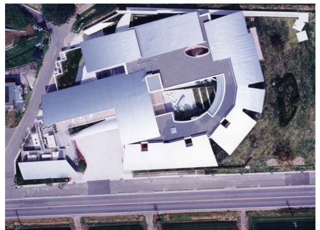
俯瞰 aerial view
